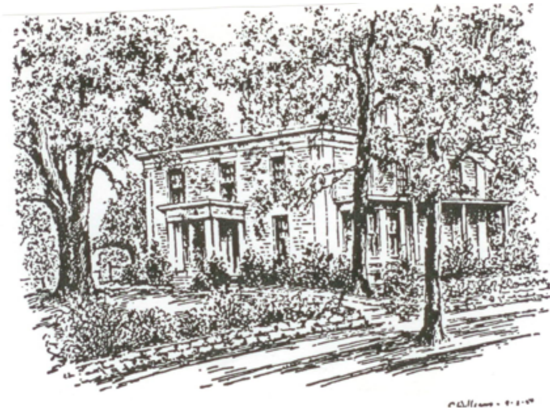
The Greek Revival style Wilson House at 1502 Aster Place
